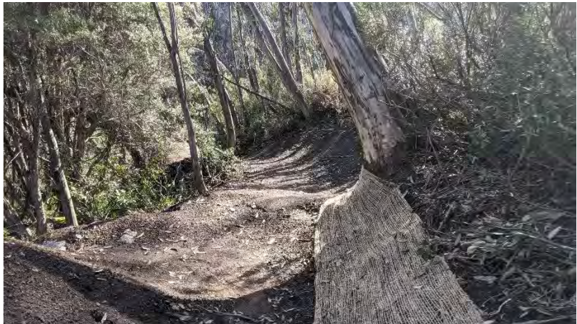
Figure 10. Example shows the trail following the contour of the slope, rather than down the fall line
